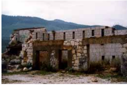
OUTER WALL OF TABIJA- NORTHERN FACADE
