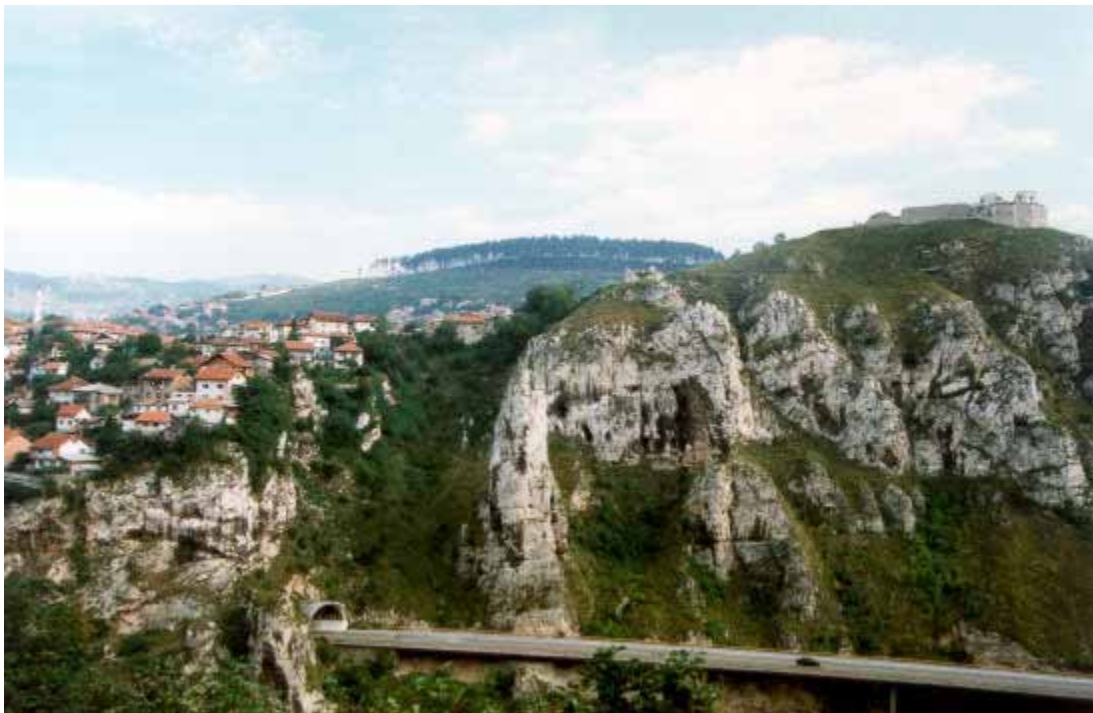
VIEW OF BIJELA TABIJA FROM THE NORTH-WEST DIRECTION
