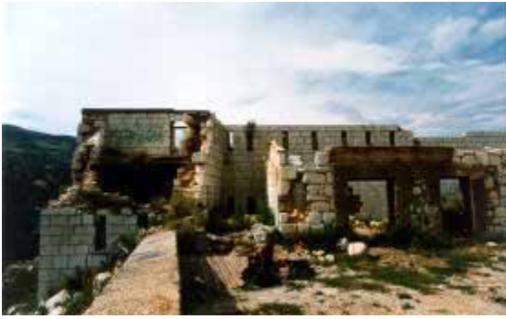
OUTER WALL OF TABIJA- NORTHERN FACADE
