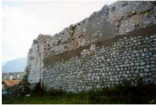
OUTER WALL - WESTERN FACADE
